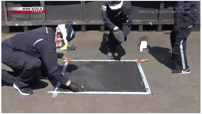
If there are a bunch of holes and it requires large scale repair work, we can lay down a temporary pavement to strengthen the road. It 's like a Band-Aid. It's a short term fix. And it 's quite effective in a disaster you may not have the means for a repair, but if you don't do something, you 'II have a collapse.
